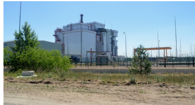
Intermediate Storage Facility (ISF-1)
