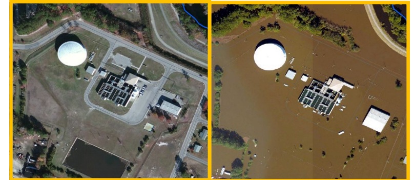
Lumberton, NC Water Treatment Plant - Hurr. Matthew in 2016
