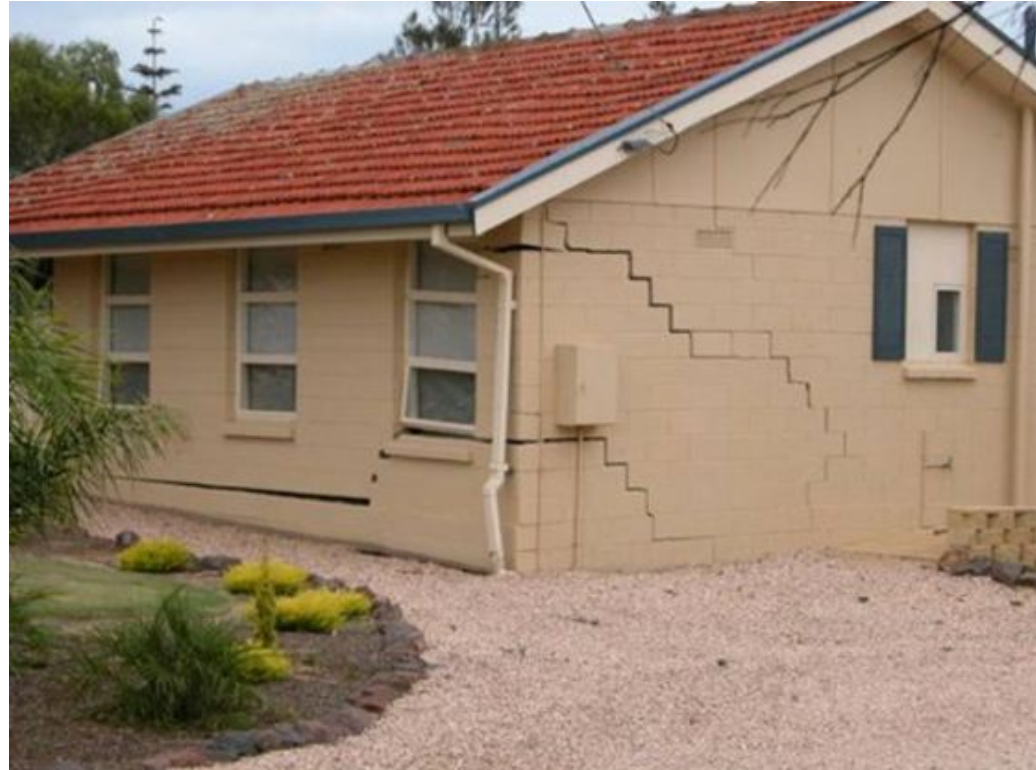
Expansive Clay Shrink-Swell
