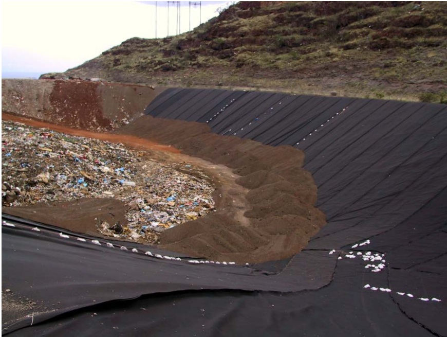
MSW landfill liner system, Waimanalo Gulch Sanitary Landfill, Oahu, HI
