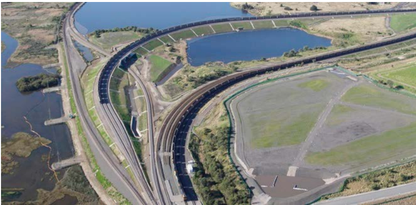
Rail Embankment Construction, Newcastle, NSW
