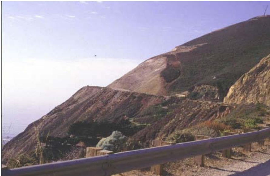
Engineered Cut Slope
