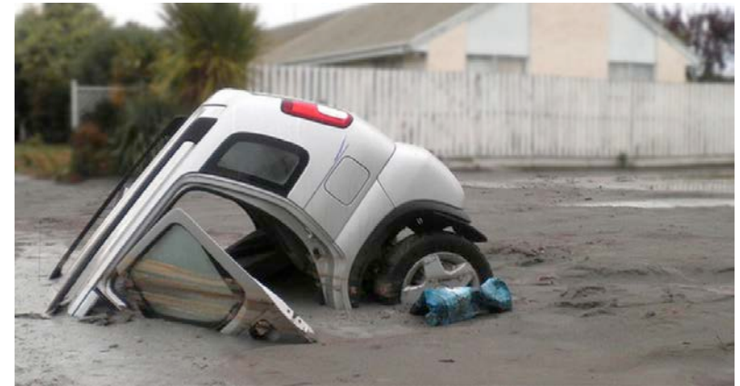
Liquefaction in Christchurch, NZ, 2011
