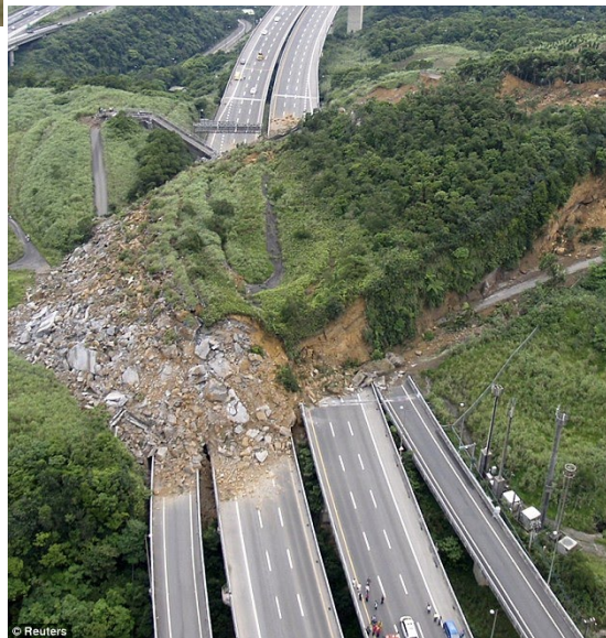
Freeway 3 Landslide, Taiwan
