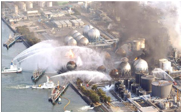
Structural Damage & Tsunamis – Fukushima, Japan
