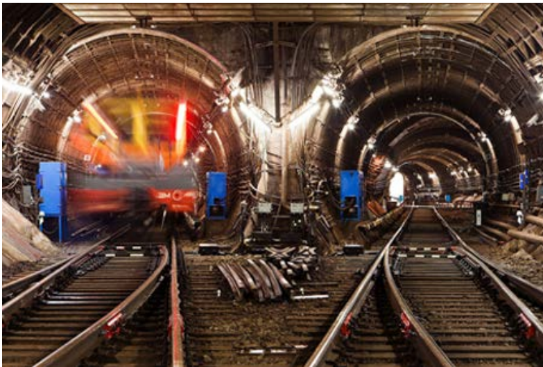
Subway Tunnel – Underground City Infrastructure
