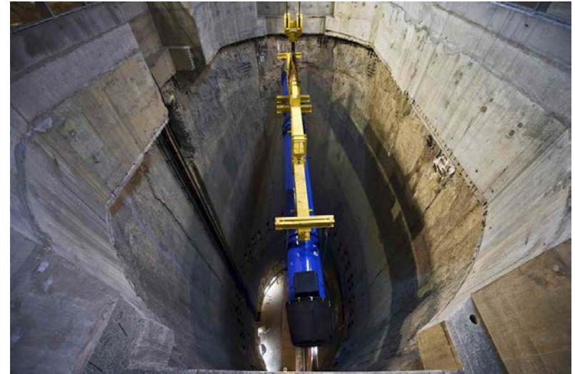
Access Into Underground Tunnel For Large Hadron Collider
