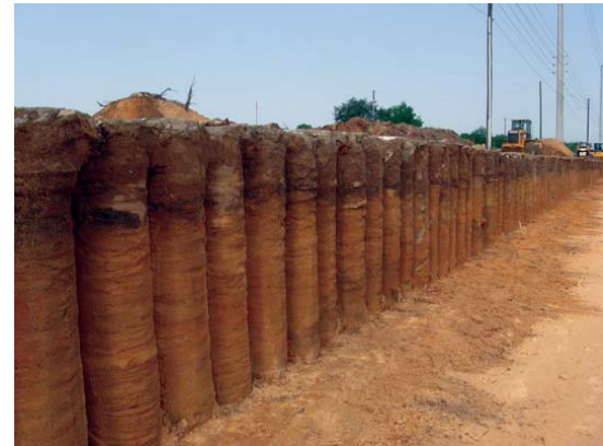
Wet Soil Mixing (Hayward Baker)
