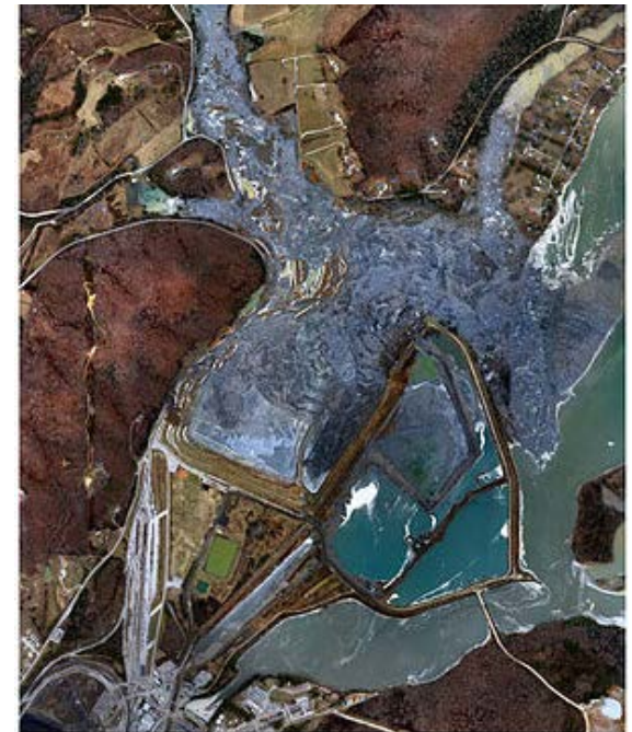
Aerial Image of Kingston Ash Slide
