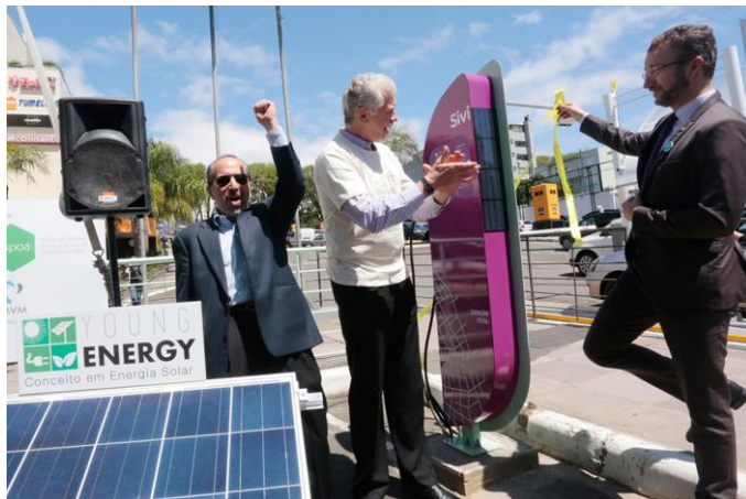
Solar Electric Car Charging Station
