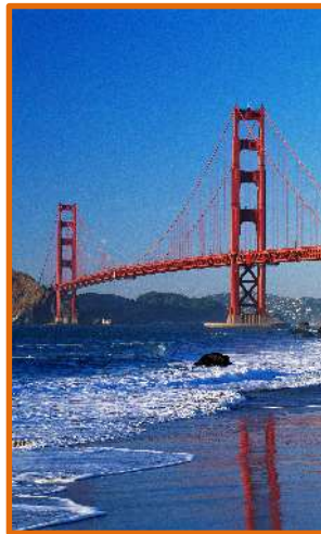
Golden Gate Bridge, CA (100 Sensors)
