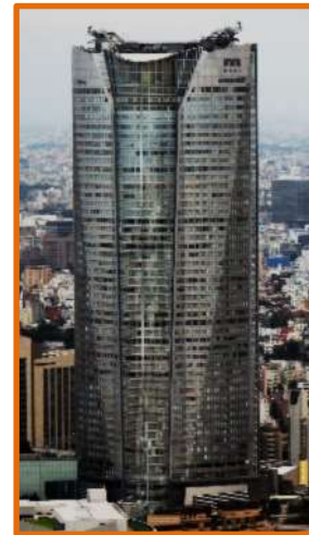
Moori Tower, Tokyo (350 Actuators)
