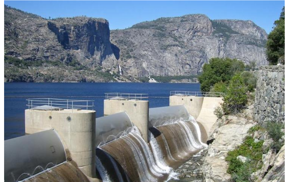
Hetch Hetchy Regional Water System forms part of the water supply for San Francisco. Photo source: Water Education Foundation
