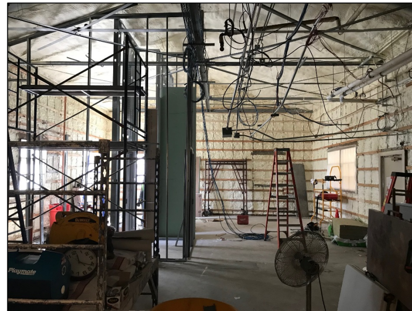
Phase 2 - Under construction (Photo date: 8/28/2018)
