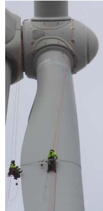
Visual inspection by rope technicians will provide commercial standard of service for blades and be used to benchmark UAV performance
