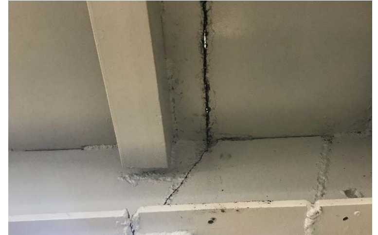
Cut main deck and supporting member
