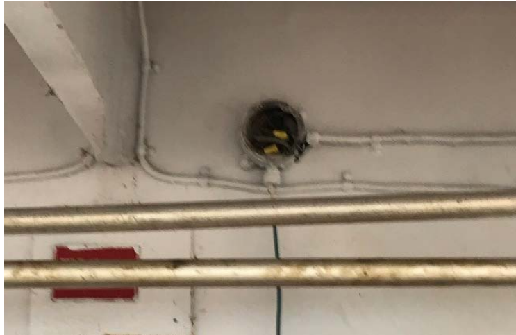
Open junction box main deck
