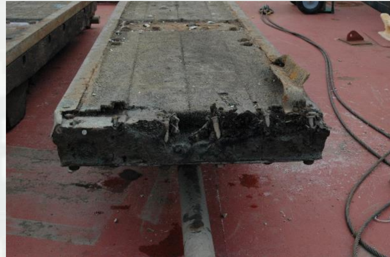
Traditional wooden wickets showing deterioration
