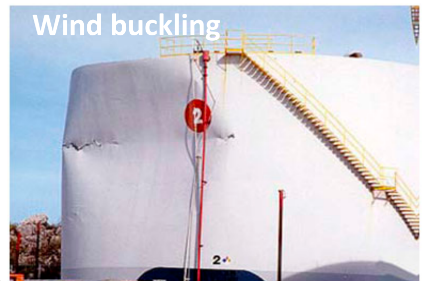
Floating roof failure
