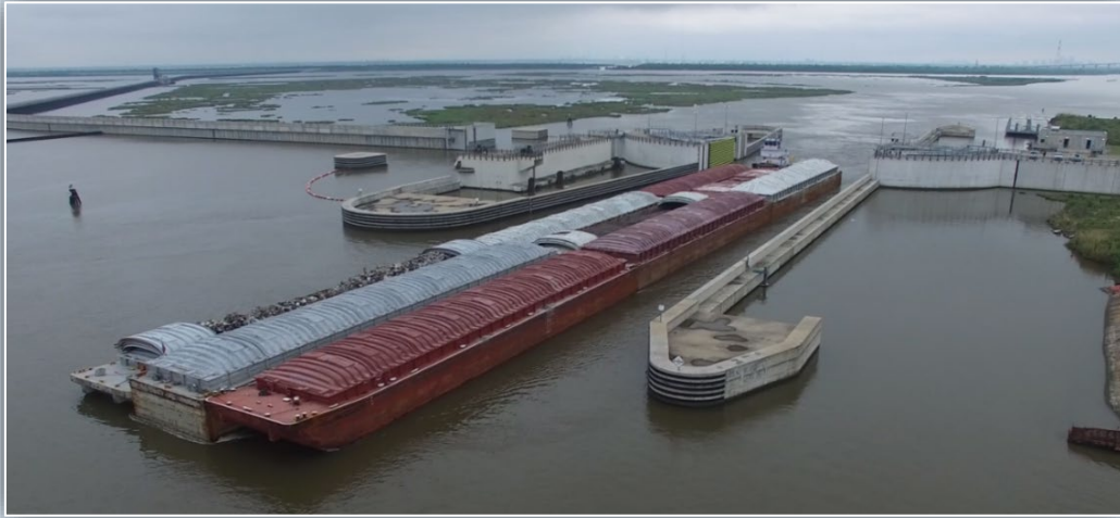
GIWW Sector Gate (150-ft.)
