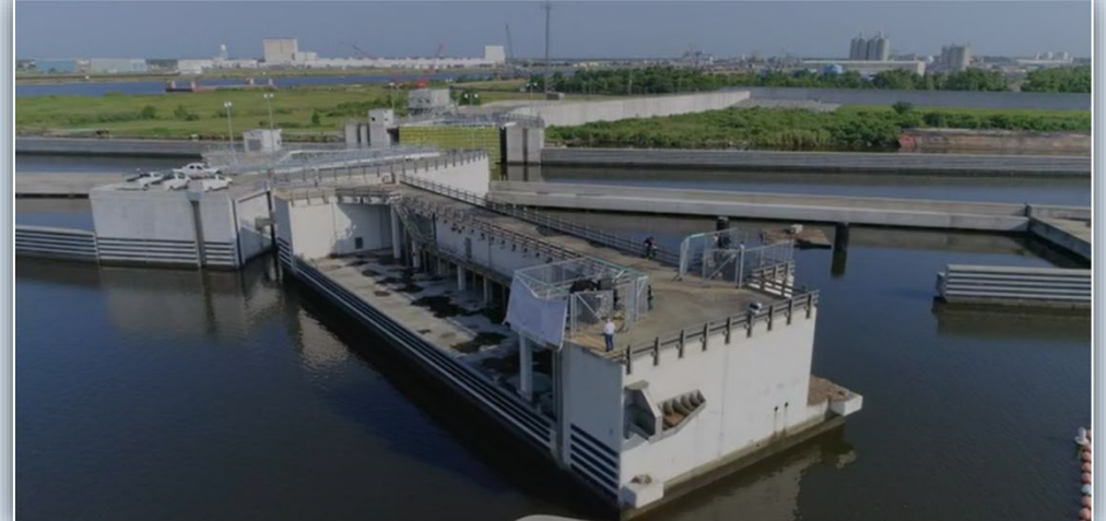
GIWW Barge Bypass Gate (150-ft.)
