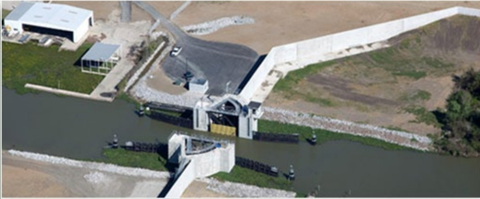
Caernarvon Control Structure (56-ft.)
