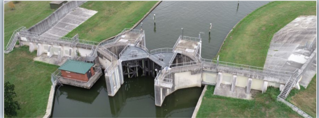
Bayou St. John Sector Gate (30-ft. non-navigable)
