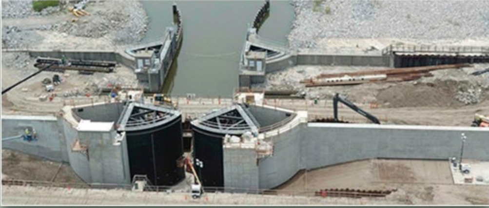
Bayou Dupre Control Structure (56-ft.)
