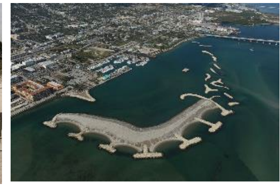
New Island Construction
