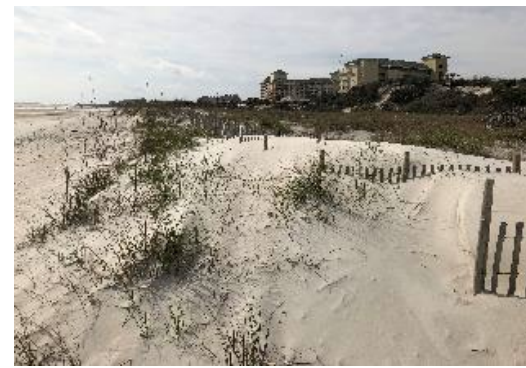
Beach and Dune Construction
