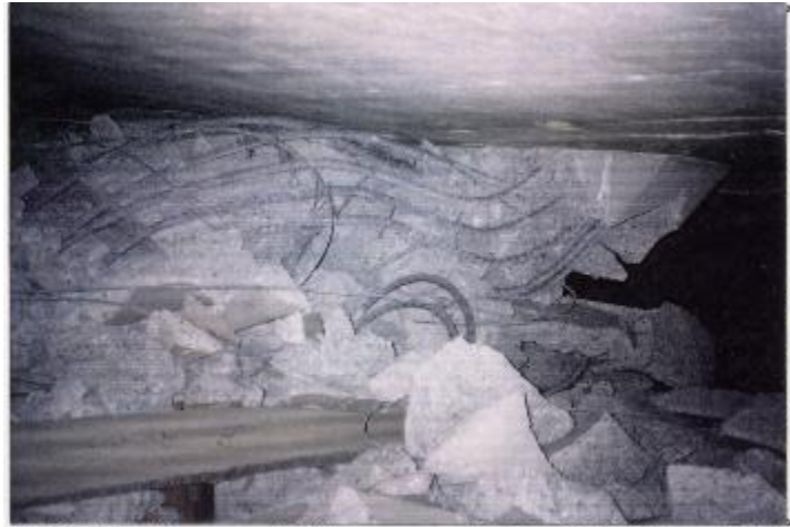
14/5 Conn. Sep. & OH Looking W @ pier 2 53-1960F 7-LA-14/5-R14.73/R45.62 1-8-BIM
