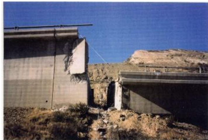
14/5 Conn. Sep. & OH Abutment #1. 53-1960F 7-LA-14/5-R14.73/R45.62 3-26-ISM
