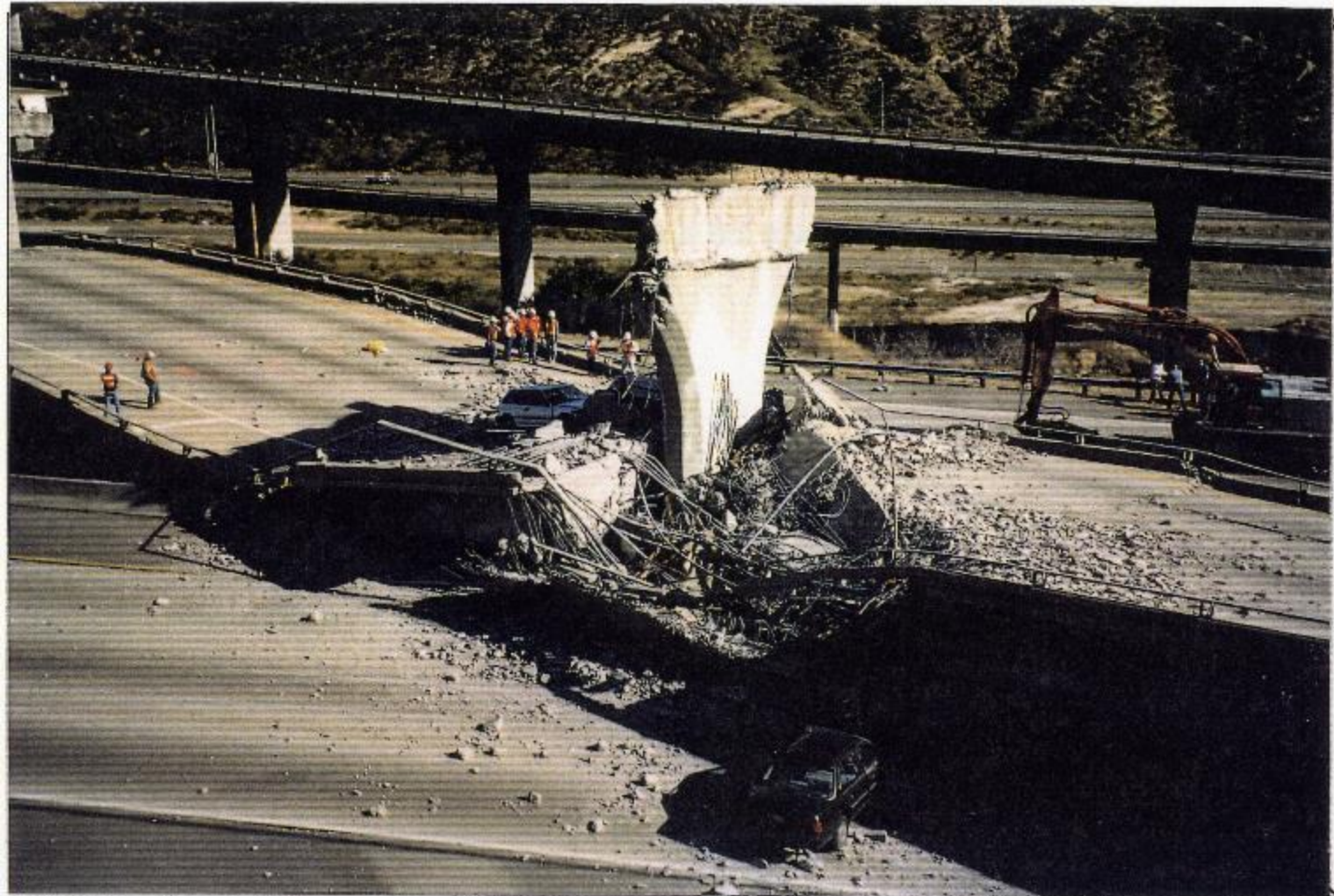
14/5 Conn. Sep. & OH Pier #3 from above, looking East
