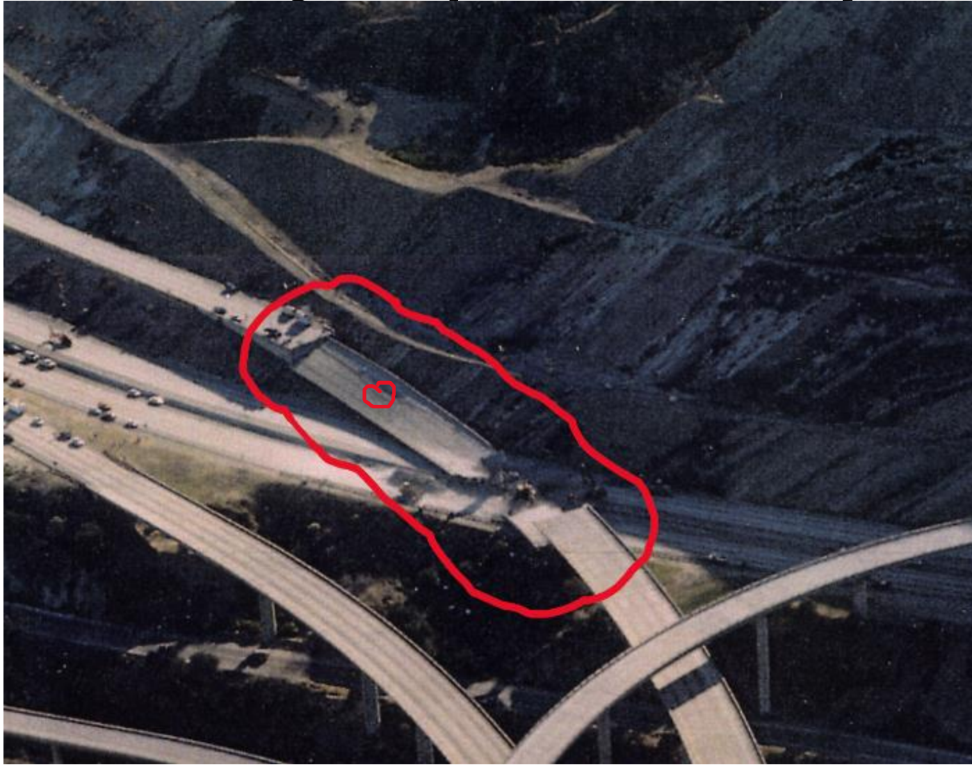
1994 Northridge Earthquake: I-5/SR-14 collapse.
