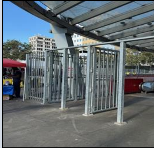
CPTED external station entrance modifications at Westlake/MacArthur Park Station. Source: David Cooper
