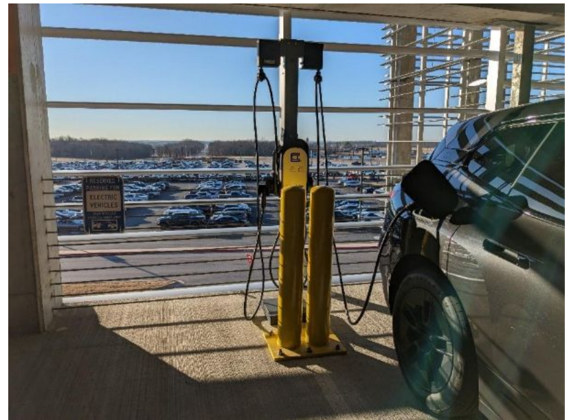
Figure 2. EV Parking Signage at Northwest Arkansas National Airport Source: Northwest Arkansas National Airport
