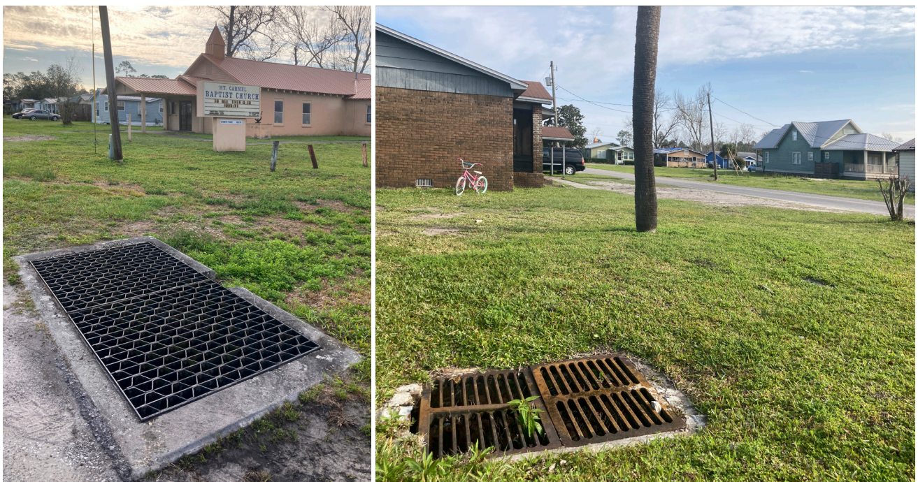
Figure 5.2. Existing stormwater inlets. In some cases inlet elevations are above surrounding grade due to land subsidence, making drainage ineffective.
