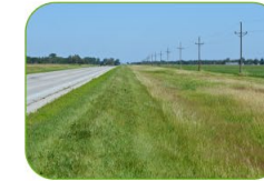
Relocation if ROW is Needed
