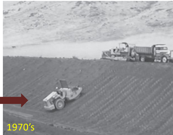
Lime Treated slope (1970's)
