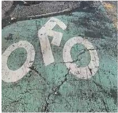
Alligator Cracking
