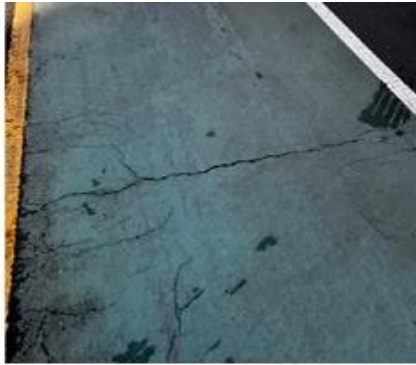
Transverse Cracking
