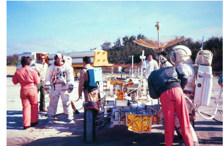
"One-G" Trainer Provided Simulation of All LRV Interfaces
