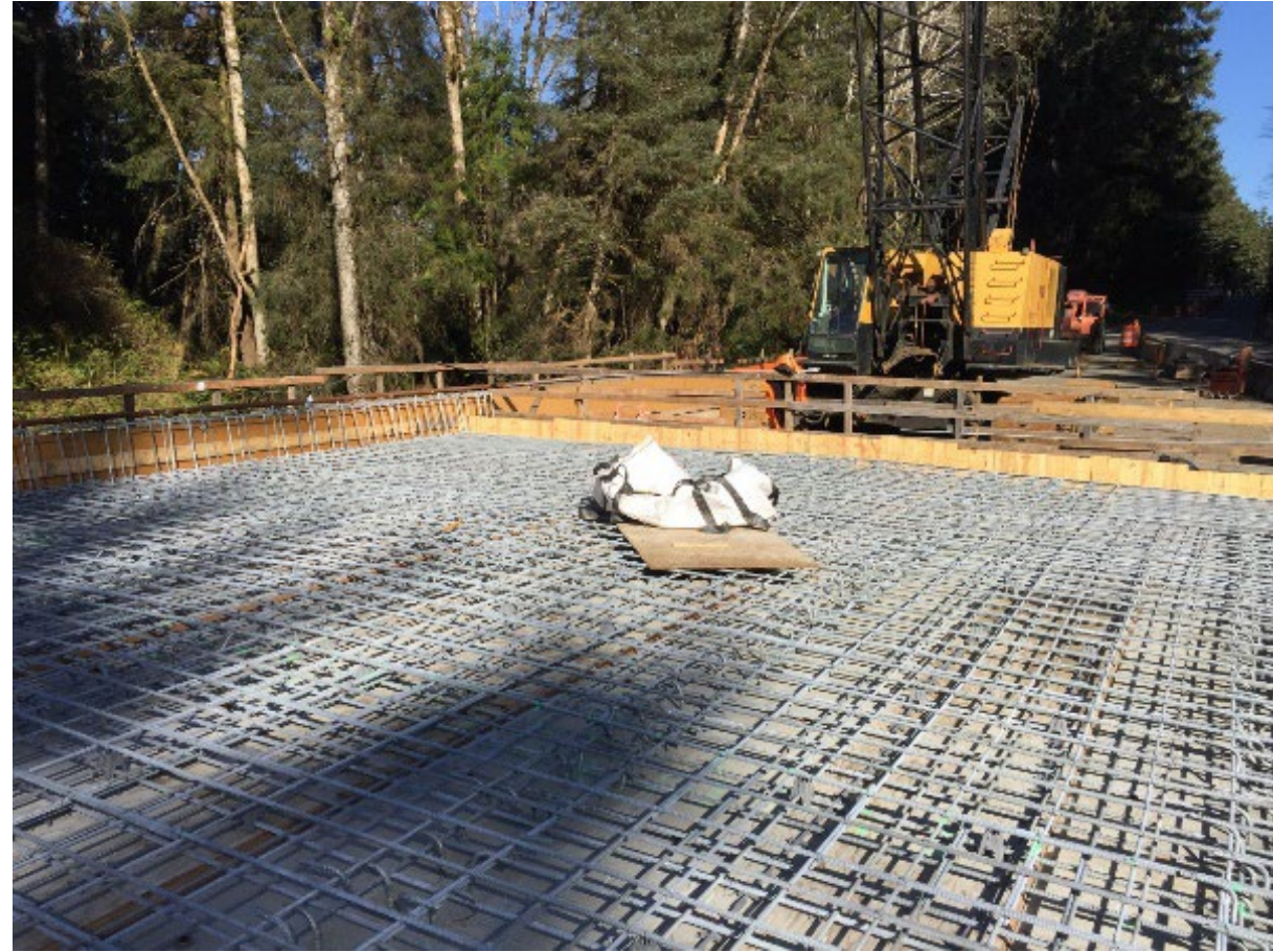
Galvanized rebar in Washington
