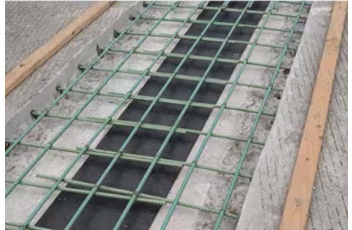
UHPC link slab from New York
