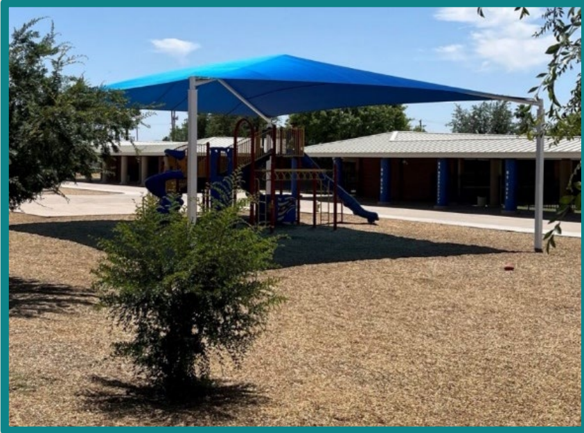
Shade structures for public transit, schools, pedestrians, and public art
