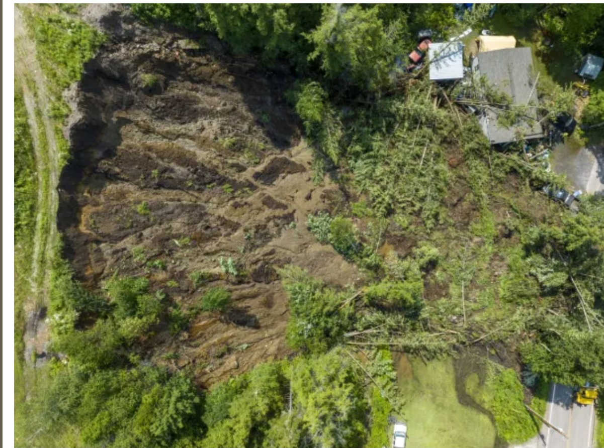
Flood damage along Route 124 in Ripon on Saturday, July 16, 2011. Photo by Caleb Koma for VTDigger.
