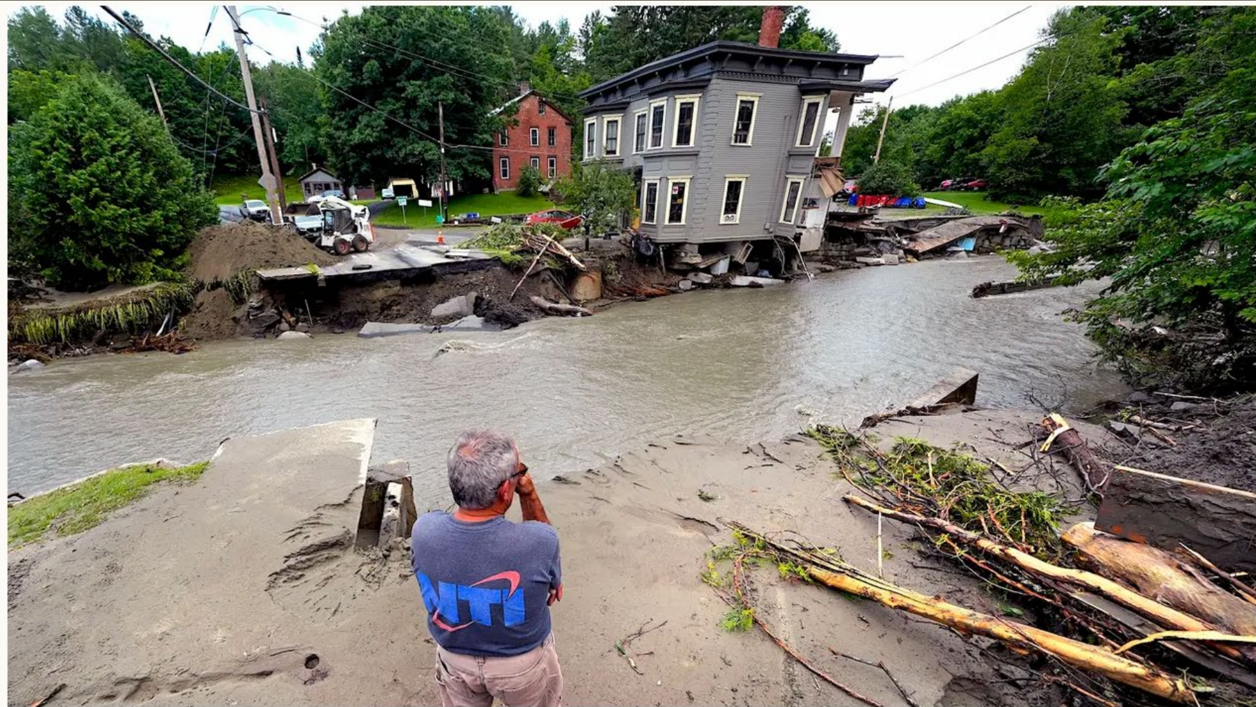
Flood damage in Plainfield, Vermont, after Hurricane Beryl, July 2024. Flooding destroyed the Mill Street Bridge and most of an adjoining apartment building. CHARLES KRUPA / AP PHOTO
