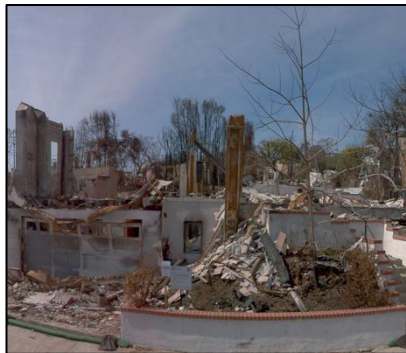
CHS Level 3: Major structural combustion
