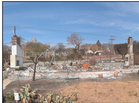
CHS Level 4: Complete combustion
