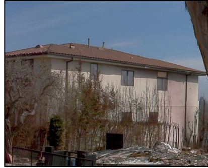
CHS Level 1: Superficial combustion
