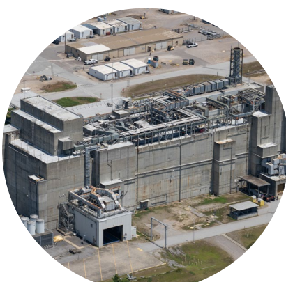
Defense Waste Processing Facility (Glass)
