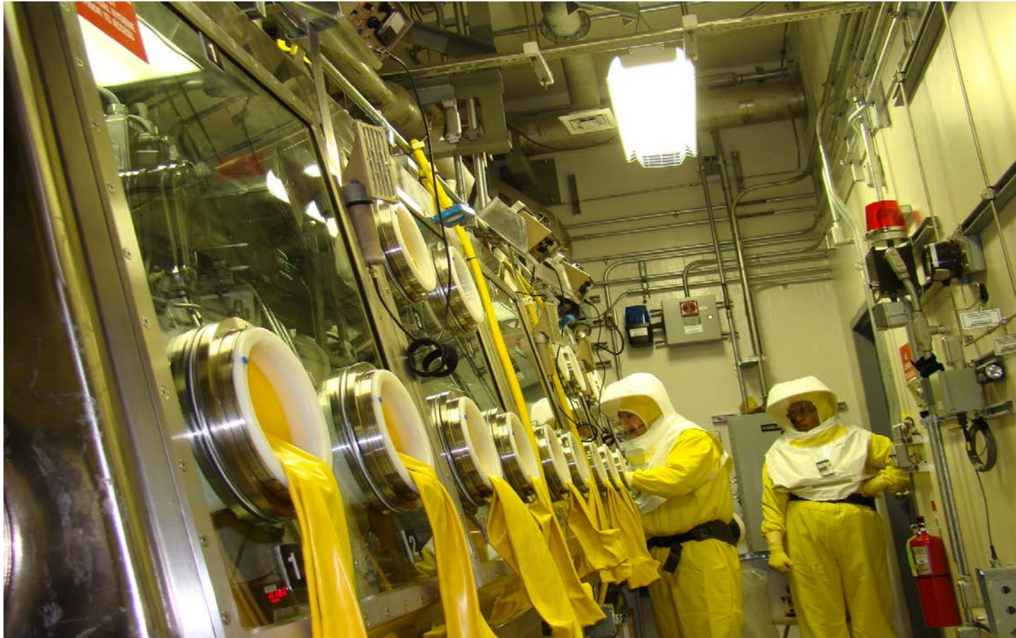
K-Area glovebox for D&D operations (from K. Fuller, Savannah River Nuclear Solutions, "Savannah River Downblending Program for Surplus, Non-Pit Plutonium, Institute of Nuclear Materials Management Annual Meeting, Atlanta, GA, July 2016
