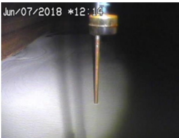
Figure L-4. Tank #34, Grout Nearing the Top
