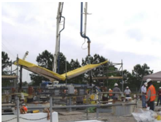
Figure L-3. Consolidated Incineration Facility Solvent Tank Grouting
