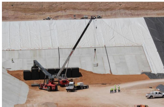
Figure G-9. Wastes Being Loaded into Modular Concrete Canisters at the Waste Control Specialists Disposal Cell
