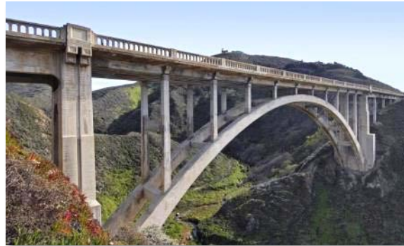
Rocky Creek Bridge
