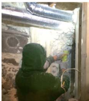
(b) Foam removal using a powered brush tool
