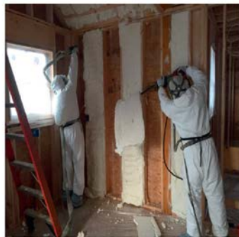
(a) Spraying and shaving of foam
