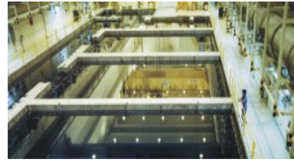
Wet fuel storage basin housing EBR-II fuel
