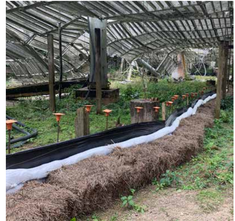
Silt fences installed for pollution prevention
