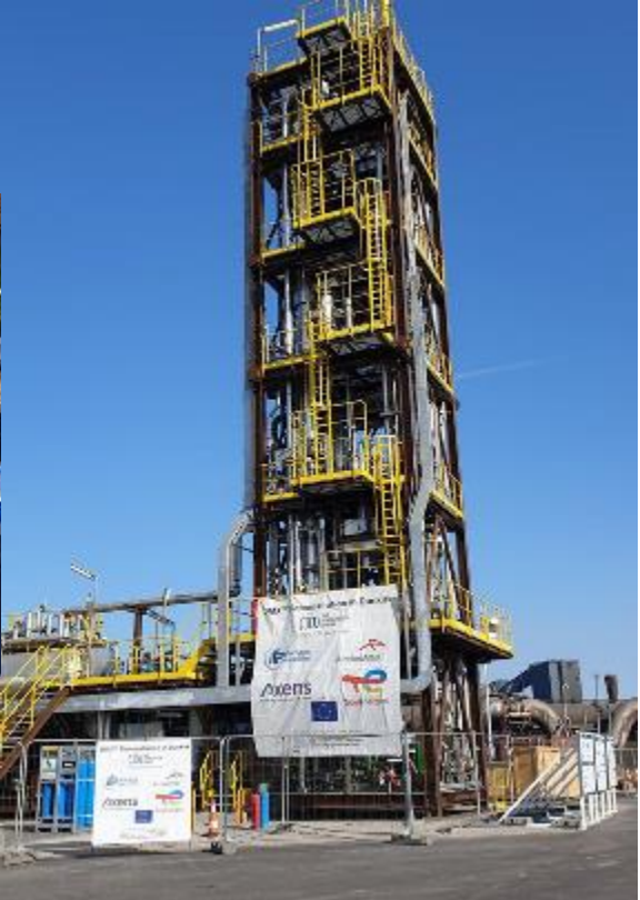
Membrane separation : AM pilot in cement plant
