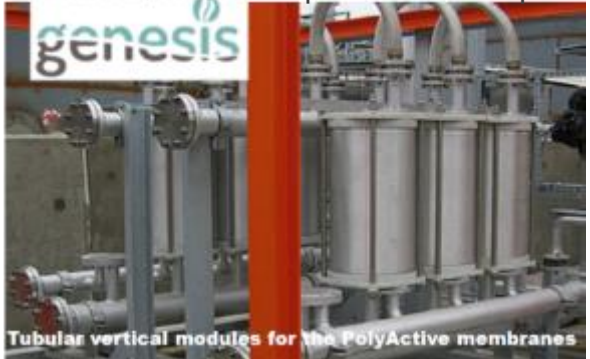
Membrane separation : AM pilot in cement plant
